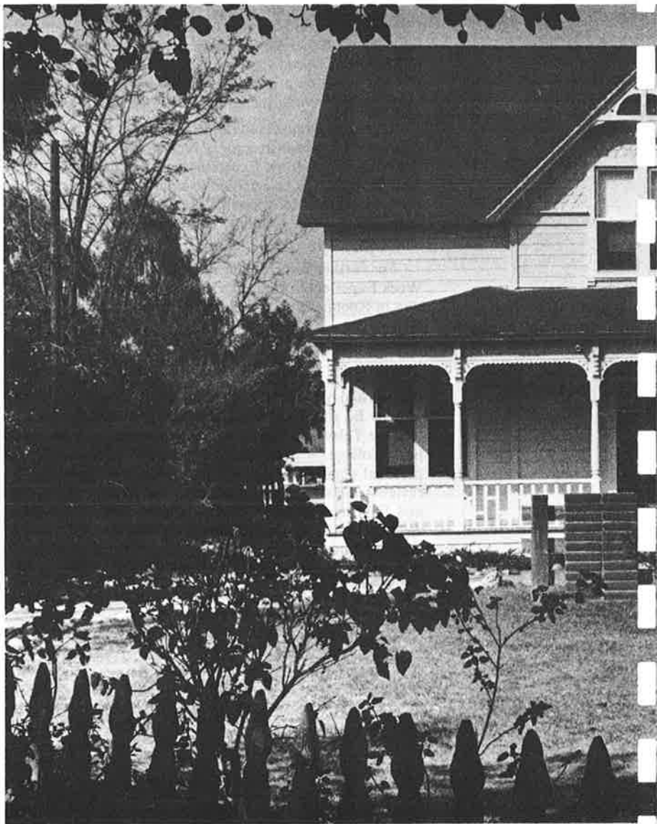
R.P. STRATHEARN HOUSE. In the 1890's R.P. Strathearn bought 14,000 acres in Simi Valley for a cattle ranch. He chose to incorporate into his new Victorian home the remains of the De La Guerra adobe which had been partially damaged by fire in the 1820's during an Indian uprising. The original adobe had been built sometime during the 1790's. The house was completed in 1903 and was lived in continuously for some 76 years. In 1969 the Strathearn family donated the 6-1/2 acre parcel of land
