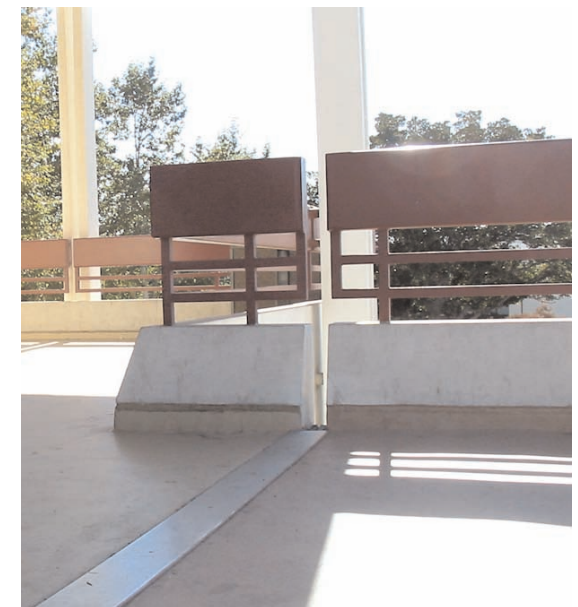
Tube steel guardrail and pre-cast detail at the second floor
