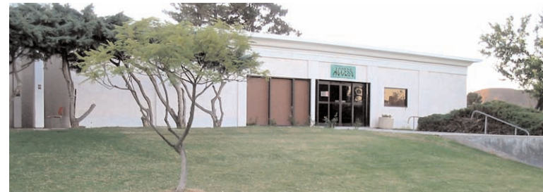
ACCESS Center exterior west facade
