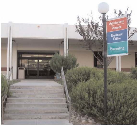
Building Administration west entrance with banners
