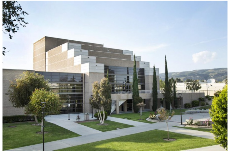
Photo the Moorpark College PAC courtesy of the VCCCD photo archive.
